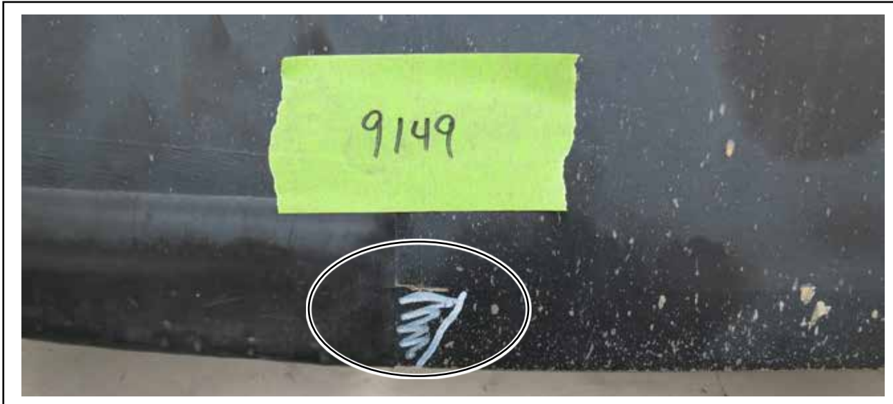
Erosion Shield Debond Figure 1-2
