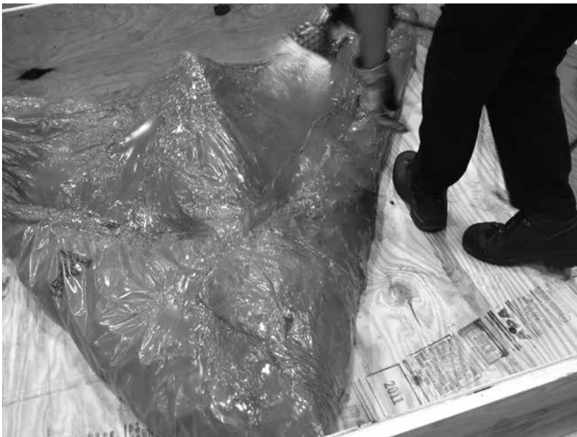
Forming a Wrap Around the Propeller Figure 3-4
